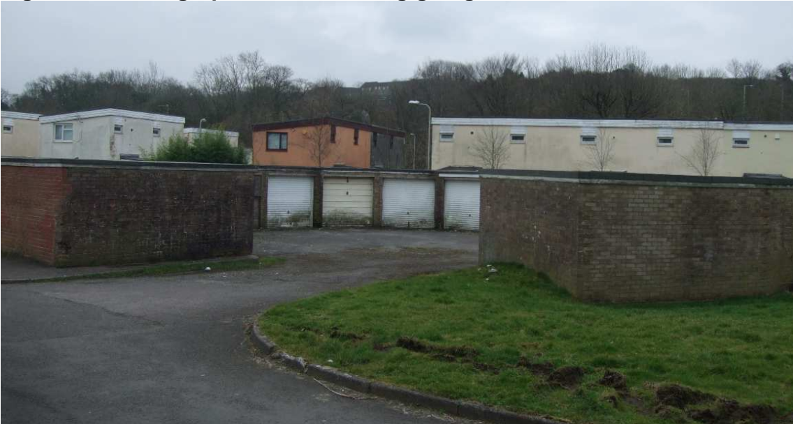
Figure 2 – Photographs of the existing garage block to be demolished.
